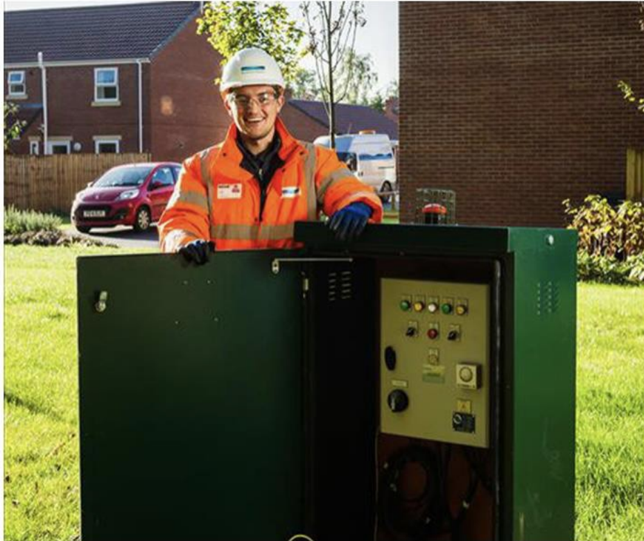
A pumping station control kiosk
